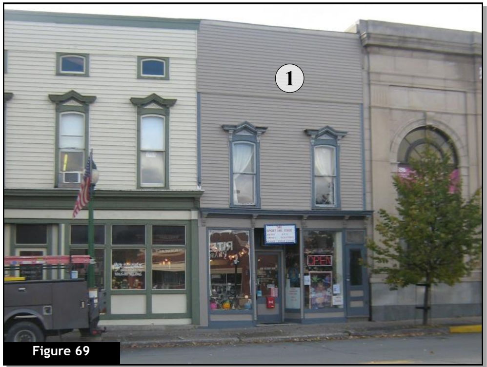
Figure 69: The use of inappropriate materials and finishes (1) diminishes the visual quality of the structure and adjacent buildings. In this example, although the structure has a high quality storefront, the use of vinyl siding over what was likely masonry construction reduces the overall appeal of the building.
