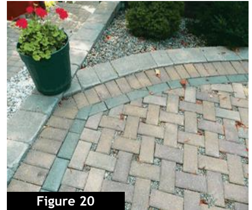
Figure 20 Porous pavements are encouraged to further facilitate infiltration and slow storm water runoff. These materials are especially useful along the periphery of parking areas and/or adjacent to bioretention areas (below).
