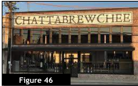
Figure 46: The contemporary modernization development seen in the above figure provides a consistent solid to void ratio and street level transparency appropriate for Main Street in Eden [F(3)(b) and (c)].
