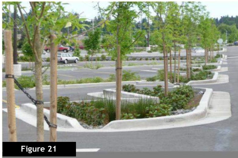
Figure 21 Where appropriate, bioretention areas and bioswales similar to the above may be used to promote the infiltration of storm water. These installations would be appropriate in parking lot medians or in linear strips along drive aisles or behind parking lots in lieu of large, unsightly retention facilities.
